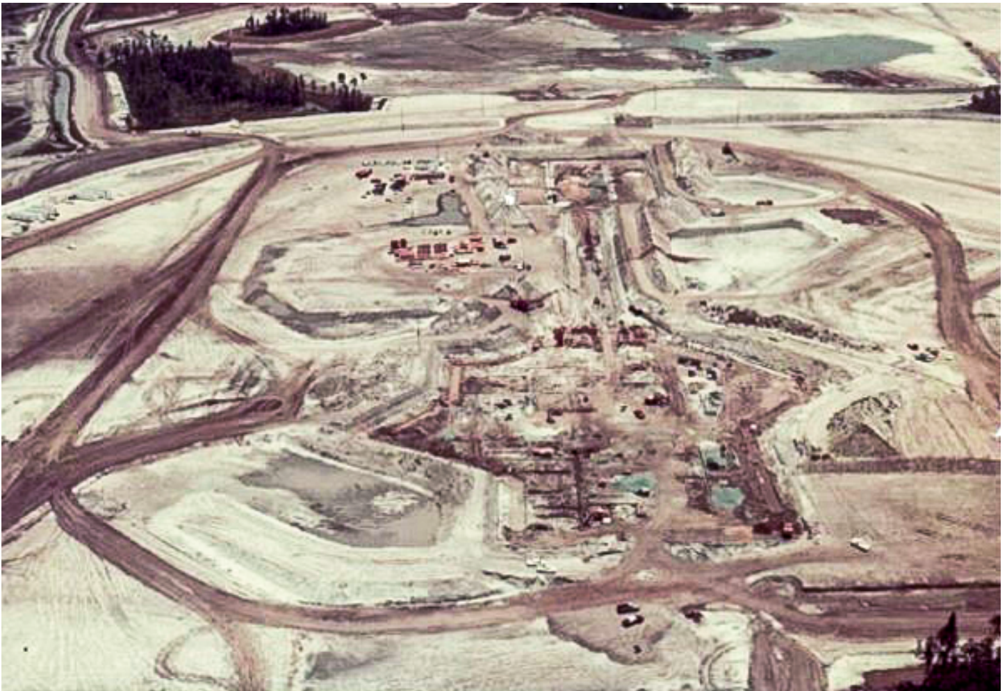
Walt Disney World Early Construction
