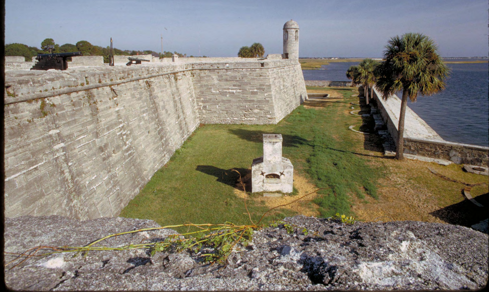
Hotshot furnace beside the seaward battlement walls at Castillo de San Marcos National Monument. National Park Service
